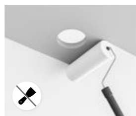
Paint the ceiling, no puttying needed
