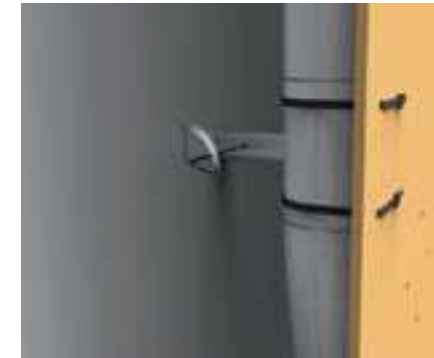
7. Detail of the wall pins fixing.
