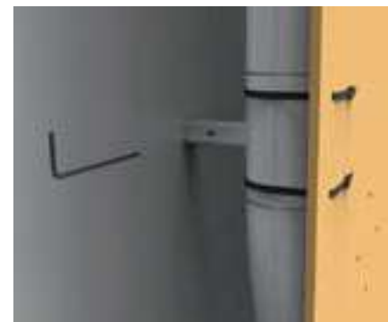
6. Detail of the wall pins fixing.
